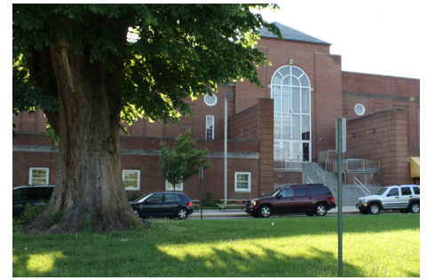
Frederick High School has a failing fire alarm system. There is but one single door opening to the outside from the lunchroom.
